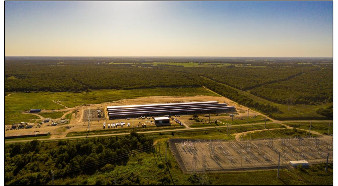
Riot Blockchain's recently announced acquisition of Whinstone U.S., a 100-acre, 750 MW Bitcoin mining facility in Rockdale, Texas
