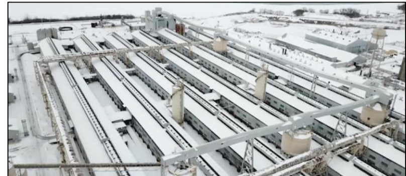
Coinmint, LLC's hosting facility in Massena, NY
